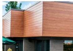
WALL PANEL #5: HORIZONTAL EXTERIOR 'OIL RUBBED' WOOD SIDING COLOR: 'MINWAX' STAIN : GUNSTOCK 231 OR APPROVED
