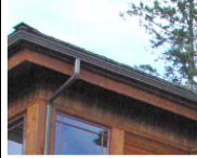
GUTTER: COMMERCIAL PROFILE MATCH ROOF COLOR - 6" SQ.
