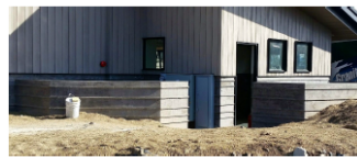
LANDSCAPE/PATIO WALLS: CONCRETE BOARD FORM COLOR: 'NATURAL' CONCRETE
