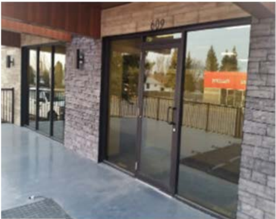
ALUMINUM STOREFRONT EXTERIOR DOORS AND WINDOWS
