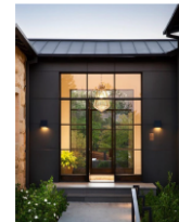
FRONT DOOR WITH WINDOWS FULL GLASS PANEL DOOR/WINDOW ANDERSON '100' SERIES/'WESTERN' OR APPR. 'MODERN STYLE', 'BLACK FRAME'
